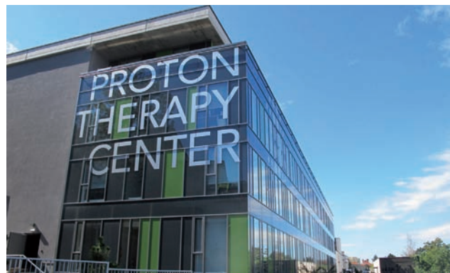
Budova PTC v Praze na Bulovce. | Foto: archiv PTC
